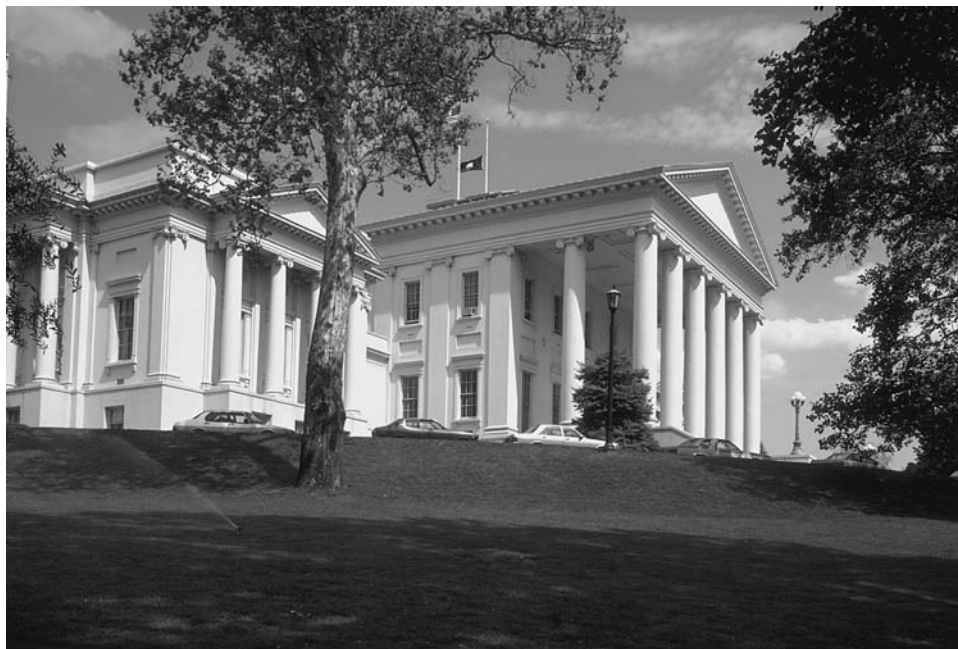
State governments are an important seat of tourism policy formation. Shown here is the state capitol building in Richmond, Virginia. Photo courtesy of Washington, D.C., and the Capital Region.
