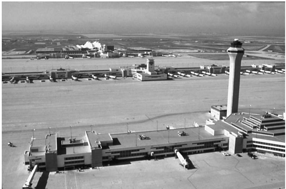
The U.S. Federal Aviation Administration provides air traffic control, air safety, and other vital aviation regulation and services. Shown here is the FAA control tower and Concourse C at the Denver International Airport. Photo courtesy of Denver International Airport.
